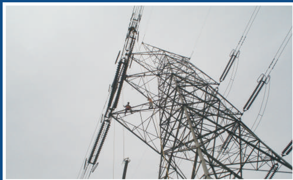
Replacement of polymer insulator in Bareilly-Mandola Section
