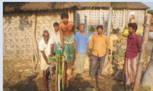
Hand pumps installed in Villages
