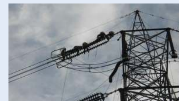
Insulator replacement work in progress on 400kV Siliguri-Purnea D/C (Quard line)
