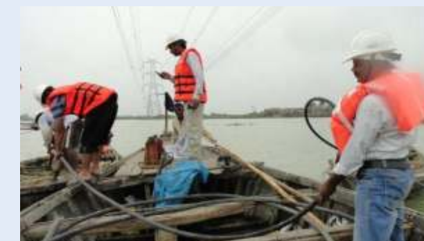
Mid-span joint replacement of 400kV Purnea - Muzaffarpur D/C (Quard line)
