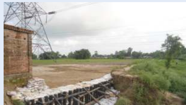
Foundation Protection of Tower No. 441 on 400kV Siliguri-Purnea D/C (Quard) line.
